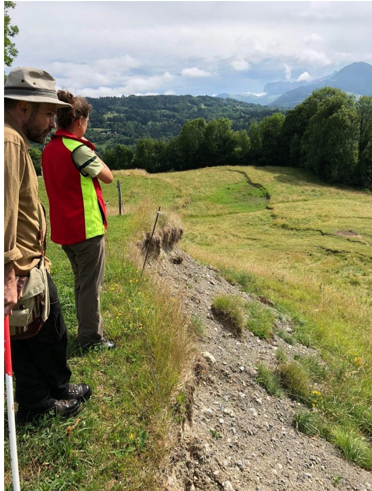
Fig.3: The head scarp of the Reyvroz landslide one year after the event © S. Justice
