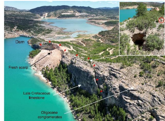
Fig.2: Active landslide located 200 m to the SW of the left abutment of the Puente de Santolea Dam (Castellote). The northern, more active portion of the landslide has been partially stabilised by removing the upper part of the displaced mass (weight reduction by beheading). The edge of the southern portion of the landslide, with limited displacement, is defined by a subvertical fissure that leads to the formation of sinkholes in the upper part of the scarp (inset, with circle indicating a dog for scale)
