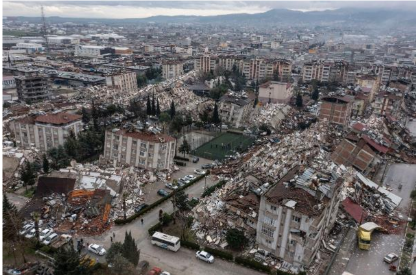
Fig. 1: Hatay city centre (Türkiye) following the February 6th 2023 earthquake in Türkiye and Syria (Photo by evrensel.net)
