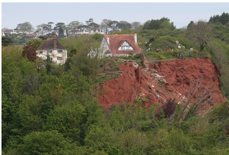
Fig.3: Upper part of the Oddicombe Landslide showing debris of collapsed house and the two other properties that are in immediate risk of collapse. Image courtesy of the English Riviera UNESCO Global Geopark (Archive Image)
