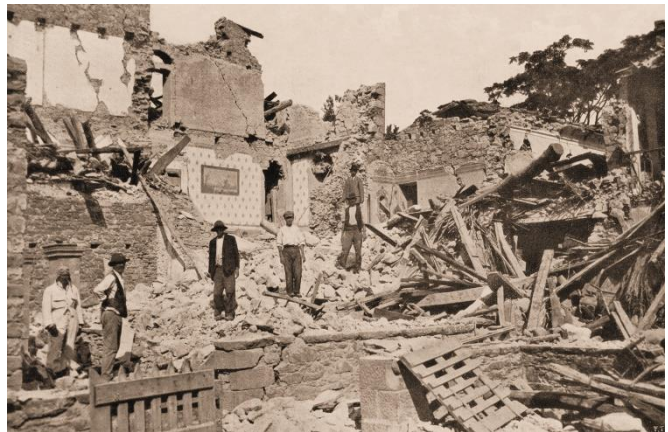
Fig.2: Collapse of buildings in the area affected by the 1920 earthquake (photo by L'illustrazione italiana, 1920)
