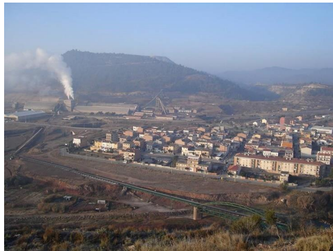
Fig.2: Estació neighbourhood before the beginning of the firsts demolitions in 2005, that lasted until 2022. (Credit: ICGC)
